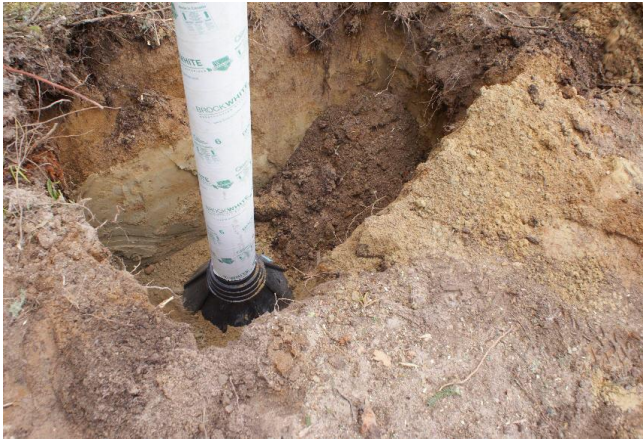
One of the supports needed for the solar panel frame.
