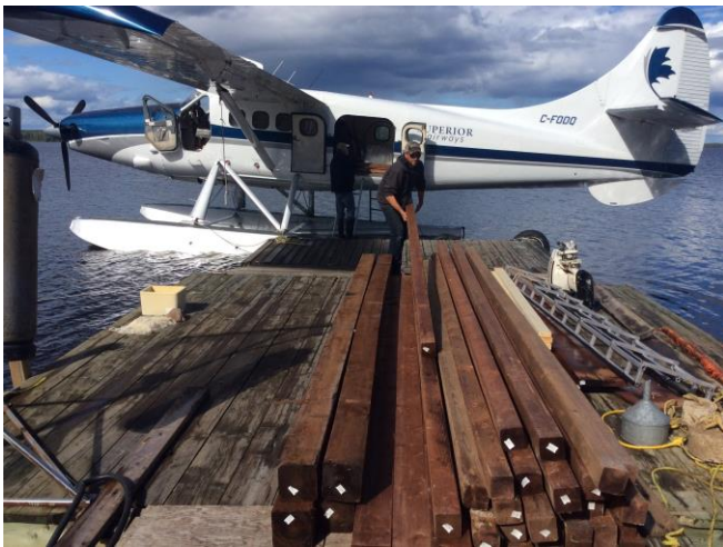
Lumber for the solar panel frame.
