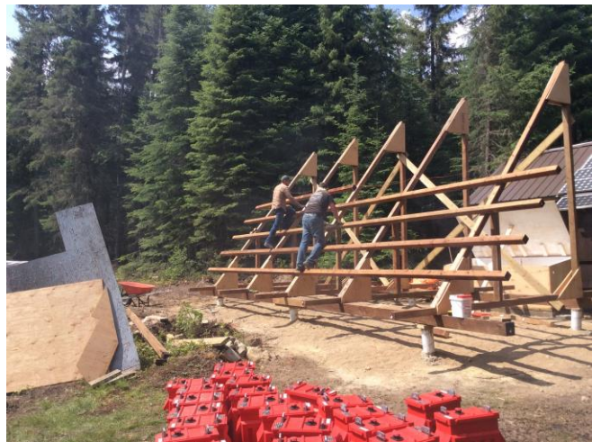
Ryan and Shaun nearing completion of the frame.
