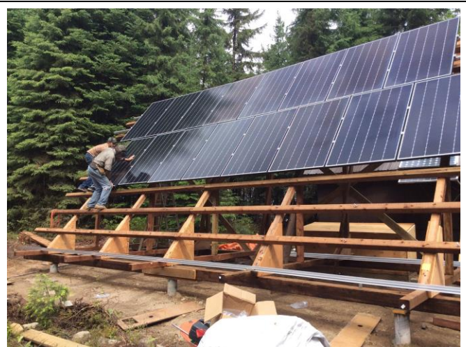
Bill and Ryan attach the solar panels to the frame.
